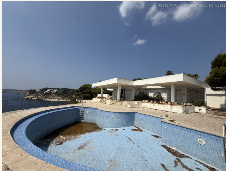
Before. Photographed from the west side of the pool terrace, 2026.
