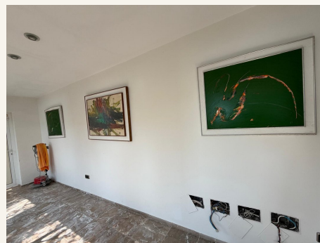
Gallery wall; services stripped back.
